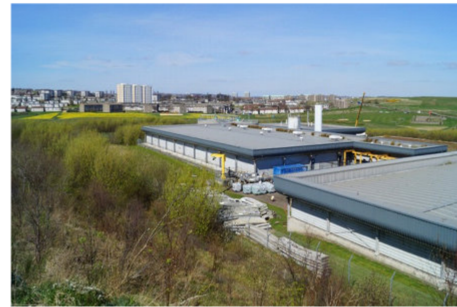
Nigg Waste Water Treatment Works
